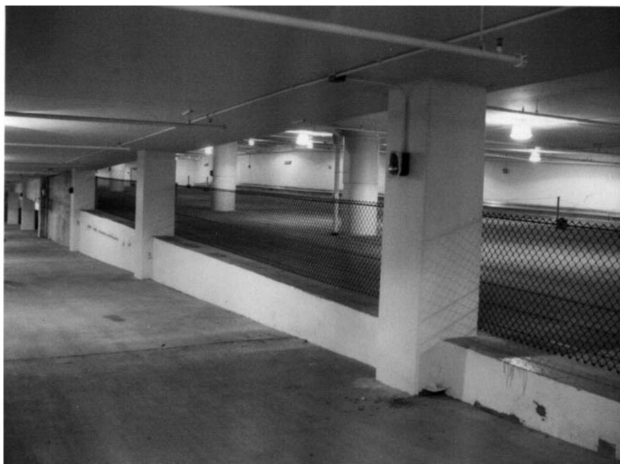
The Interior of The Garage
