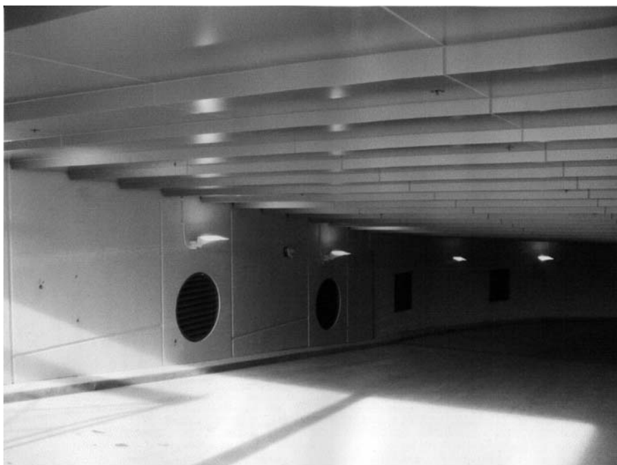
The Interior Garage Ramp
